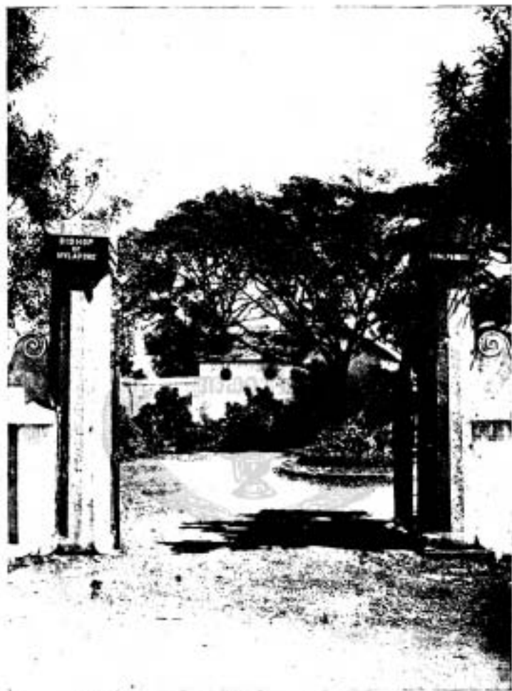
Two monolithic pillars (A 48a, A 48b) at the entrance to the garden of Bishop's House, San Thomé High Rd. Cf. p. 16, No. 15.
