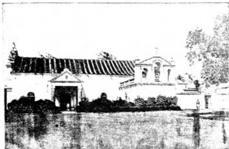
S. Thomé.—The Old Cathedral, pulled down in 1892.
